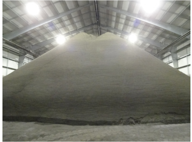
Birchwood ADOT Interior sand storage
