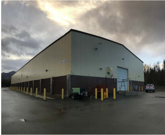
Anchorage ADOT sand storage facility
