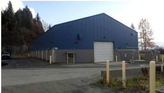
Girdwood ADOT sand storage facility
