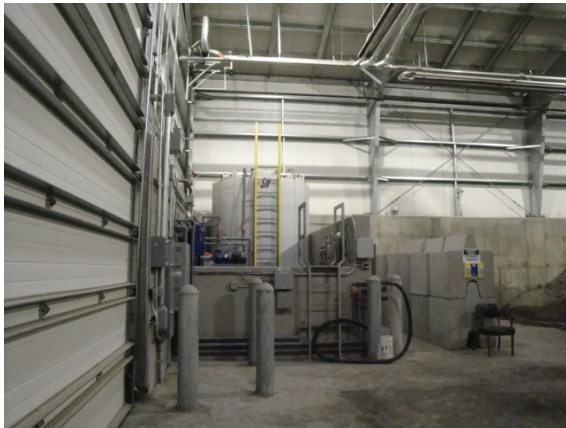
Birchwood ADOT sand storage
