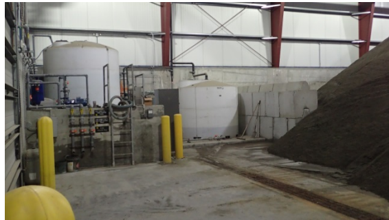
Girdwood ADOT Interior sand storage facility
